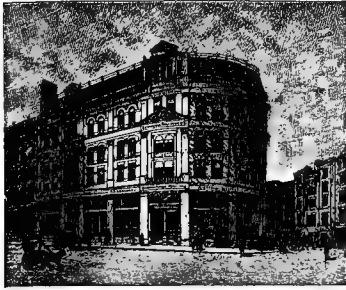
B., W. & Co.'s Offices & Warehouses, occupying Seven Floors in all.
